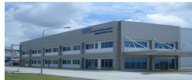
SEI Thai Electric Conductor Co., Ltd.
