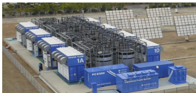
Redox Flow Battery
