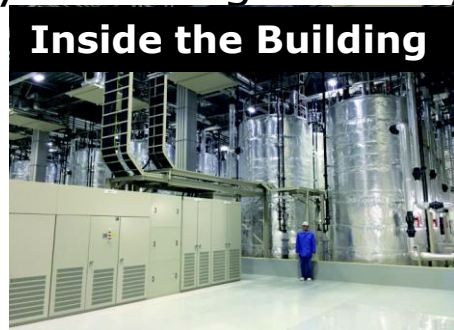
Hokkaido Electric RF Battery Building
