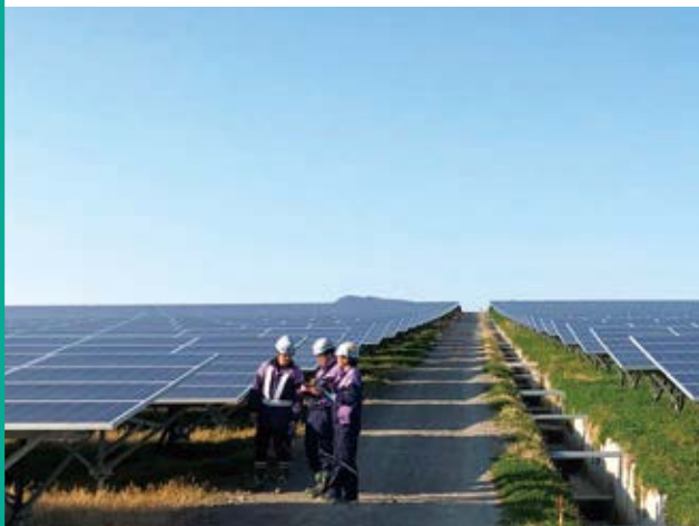
Construction work of a mega-solar system
