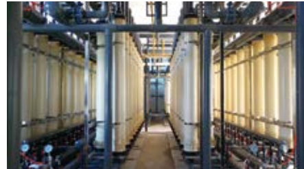
Sumitomo Electric's water treatment membrane modules delivered to Wastewater Treatment Plant in shipan town, Jianyang City, Sichuan Province
