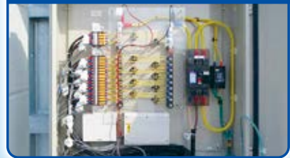
Power Line Communication (PLC)
