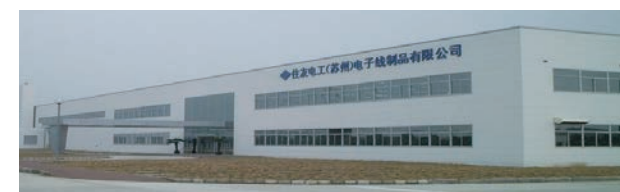
The China Analysis Technology Center is located in the Sumitomo Electric Interconnect Products (Suzhou) Ltd. (SESZ) building.
