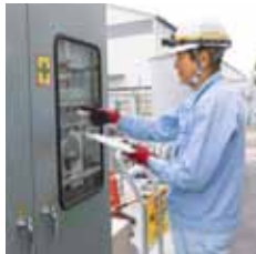
Inspection of the operational status of the system
