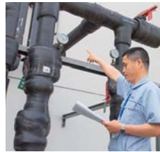
Adjustment of the pressure of cooling water
