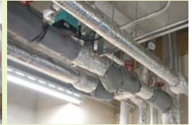
Thermal insulation of steam pipes
