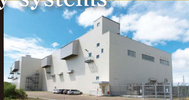
Building housing the storage battery system
