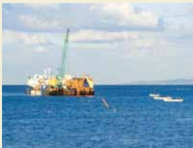
Submarine cable laying
