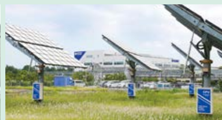
Concentrator photovoltaic (CPV) system
