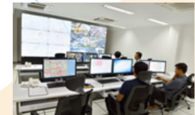
Traffic control systems These systems collect and analyze a wide range of transport information and use it to control traffic lights and provide transport information, enabling a safe and smooth flow of traffic.
