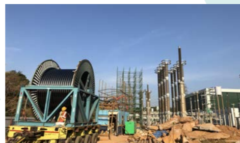
Cable installation site in India
