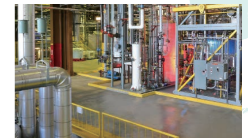
Plant in NY, U.S.A. with recycling system
