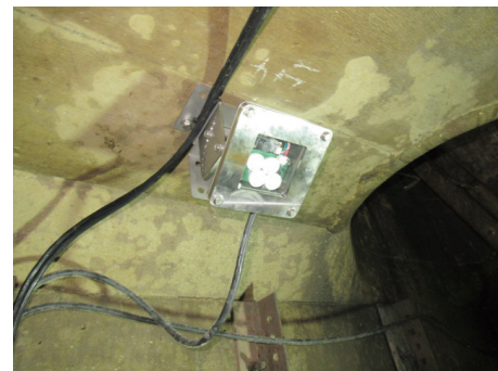
Photo 2. Example of camera installation in manhole
