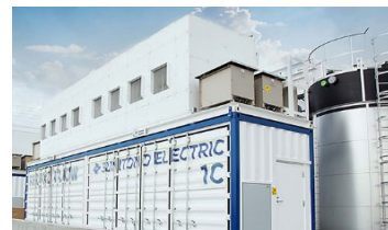
San Diego Gas & Electric in USA
