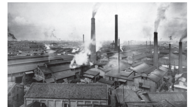
View of the entire Sumitomo Copper Rolling Works at Ajigawa (photo supplied by Sumitomo Historical Archives)
