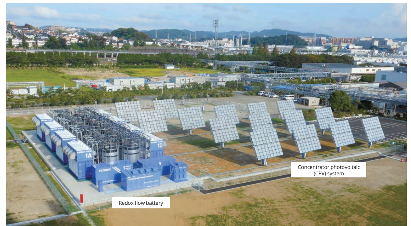
Demonstration project of a large-scale power generation/storage system (Yokohama Works)
