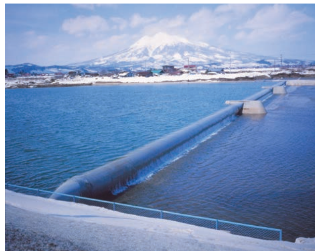
Iwakigawa intake weir Fabridam
