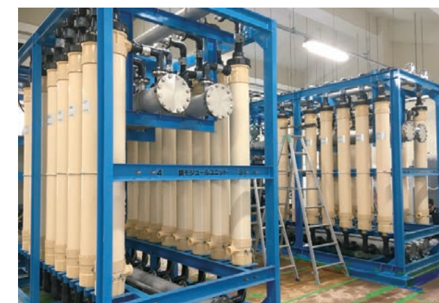
Pressurized module for wastewater treatment
