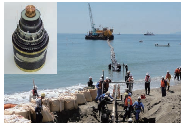
Construction of the Hokkaido-Honshu (Kitahon) HVDC Link
