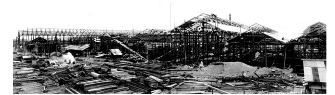
Construction of Okijima Plant
