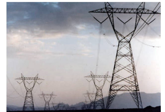
Transmission line construction in Iran
