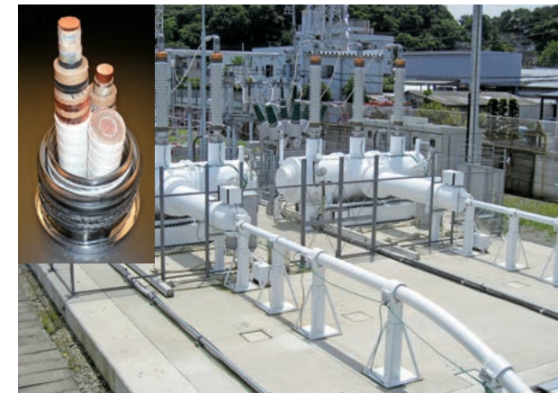
Superconducting cable project
