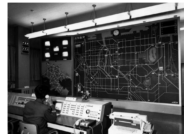
Japan's first wide-area traffic control system (Fukuoka Prefectural Police Headquarters)
