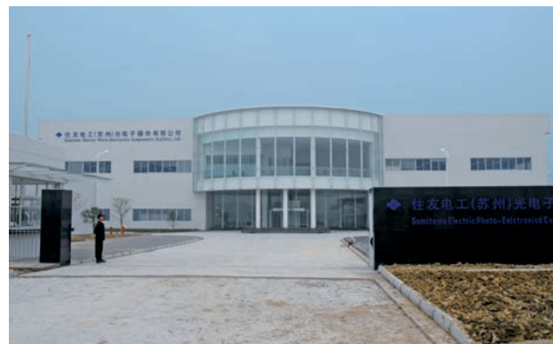
Sumitomo Electric Photo-Electronics Components (Suzhou), Ltd.
