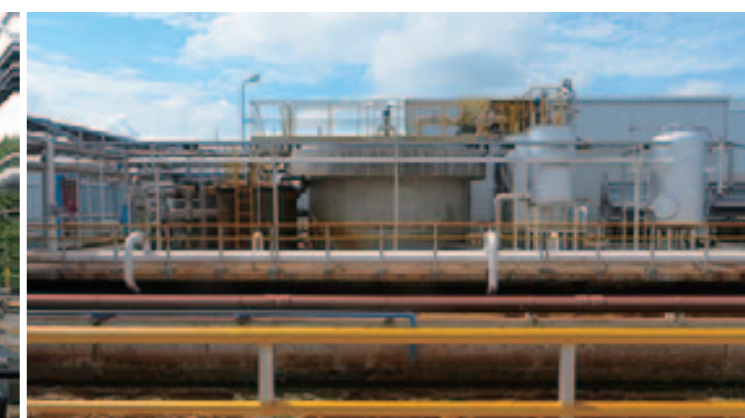
Wastewater treatment system installed in the Thailand Plant
