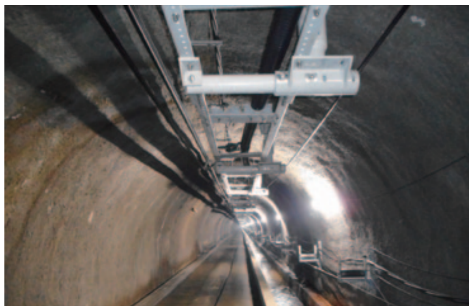
After being pulled into the tunnel, the cable is placed on supports mounted on the ceiling.
