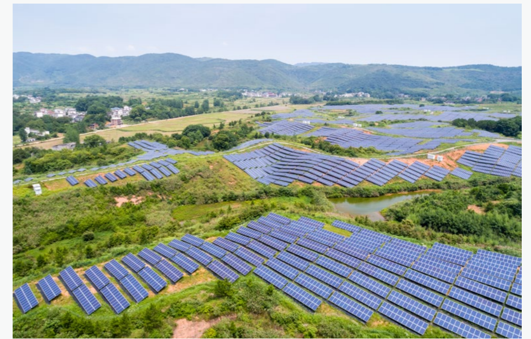
Abnormality detection is difficult in photovoltaic power plants where many photovoltaic panels installed in a large area are in operation.
