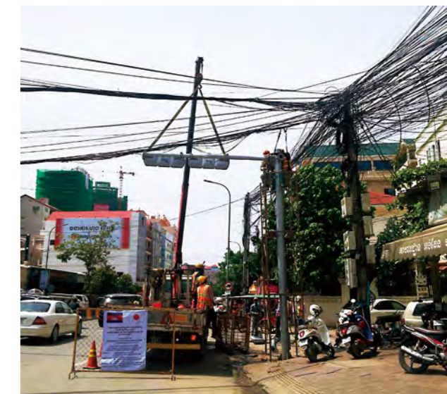
▲ Construction was proceeded by unraveling tangled electric cables
