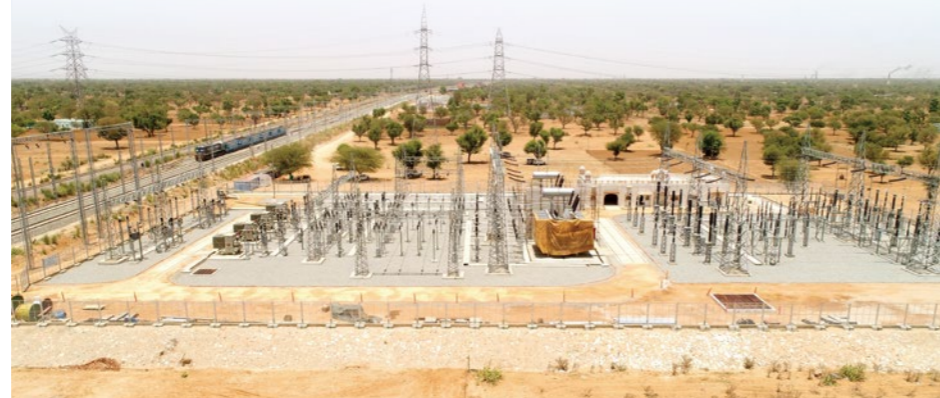
Substation built in a desert beside a railroad; To ensure stable power supply, substations are built equidistantly within a total distance of 1,500 km.
