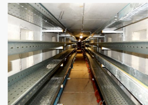
MCF-equipped underground tunnel in city of L'Aquila
