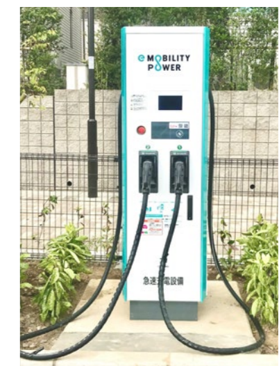
S-FREE™ traveling cable for charging EVs
