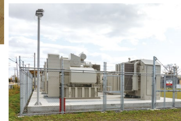
Grid connection switching station
