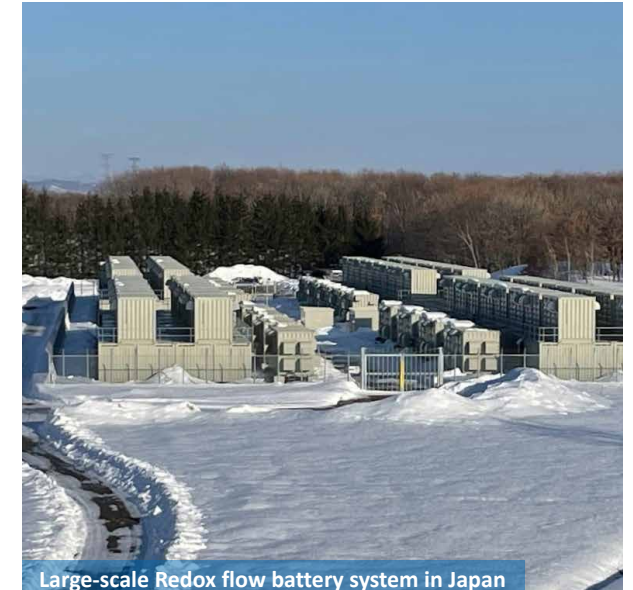
Large-scale Redox flow battery system in Japan
