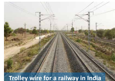
Trolley wire for a railway in India
