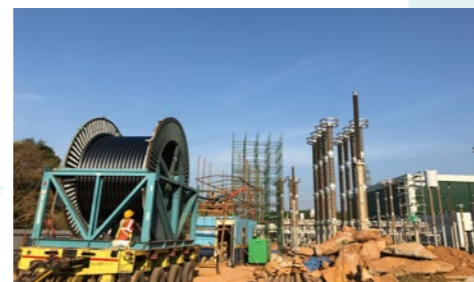
Cable installation site in India
