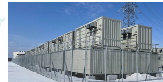
Redox flow battery system for Hokkaido Electric Power Network, Inc.
