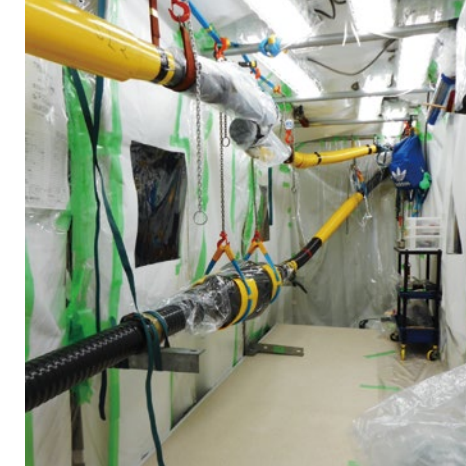
Cable connection room: Workers made efforts to implement dustproof measures in the severe environment.
