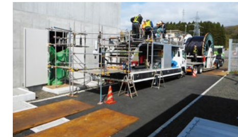
Installation (on the Hokkaido side: Yoshioka cable head (draw-in port))
