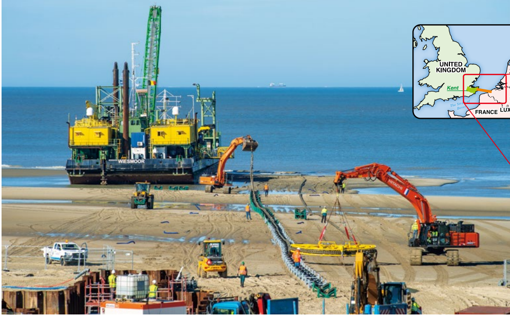
Cable laying on the Belgium beach side
