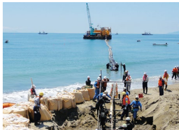
Cable installation for the Hokkaido-Honshu HDVC Link
