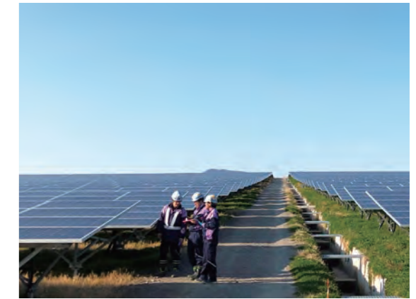
Construction work of a mega-solar system
