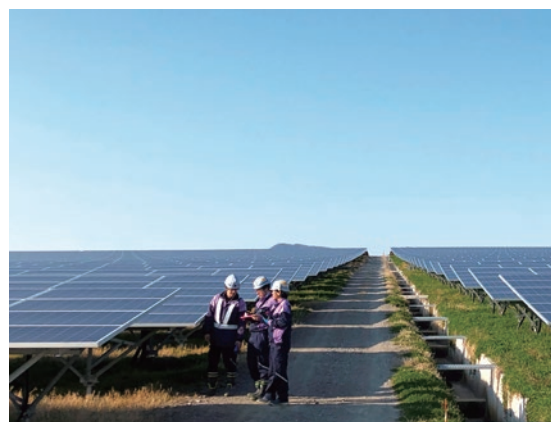
Construction work of a mega-solar system
