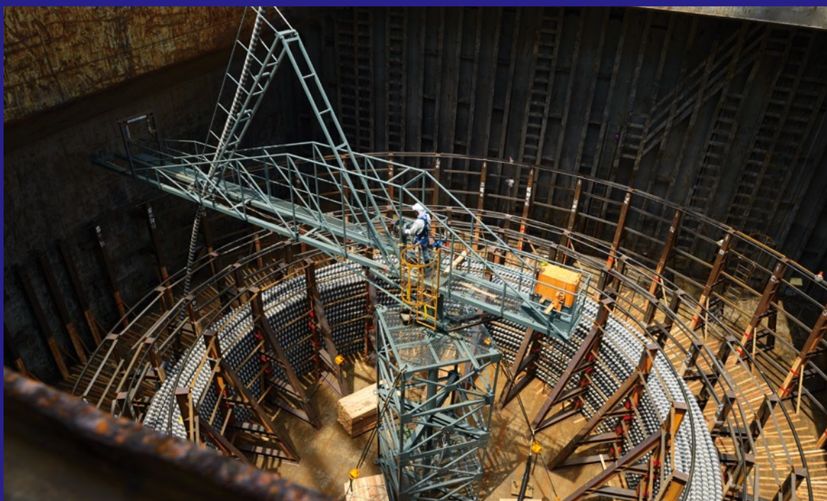
DC XLPE insulated cables loaded onto the freighter to NEMO Link
