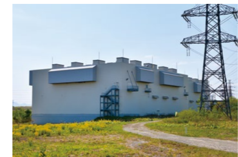
Energy storage battery building
