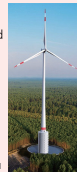
Tower for wind-power generation
